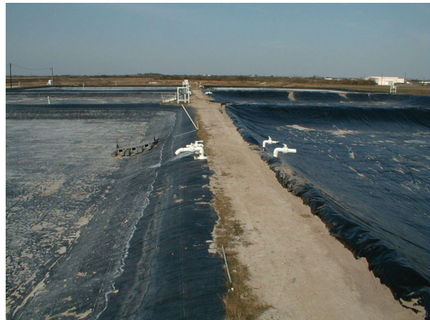
Figure 8: Open ponds often use pond liners to limit water discharge and prevent contamination of culture medium. Source: AgriLife Research Mariculture Laboratory, Flour Bluff, Texas.
