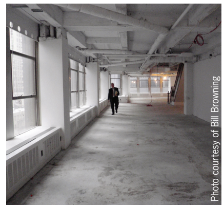
675 Third Avenue includes perimeter induction units, single-glazed curtain wall, and overhead ductwork that limits floor-to-ceiling height.
