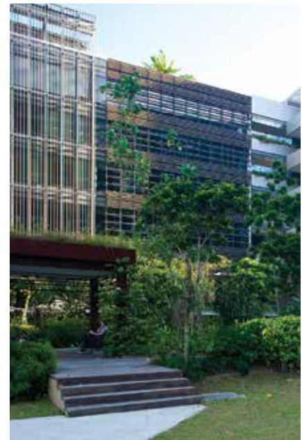
Above: The Khoo Teck Puat Hospital in Singapore by RMJM Architects uses fresh air and sunlight to increase thermal comfort. Image © Jui-Yong Sim/Flickr.
