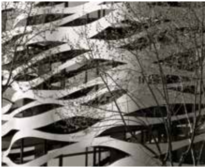
Façade renovation of Suites Avenue Aparthotel by Toyo Ito, Barcelona, Spain, is biomorphic in form, while enhancing the Dynamic & Diffuse light and shadows filtering to the interior space. Image © Aslaj/Flickr.
